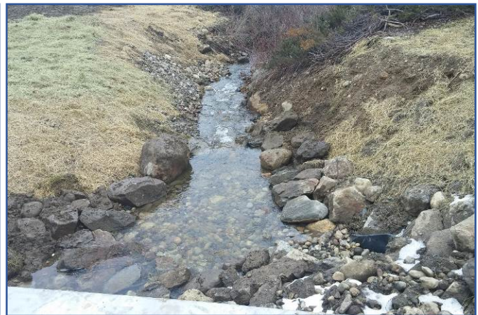
Right. Restored stream channel immediately downstream of the Route 118 culvert.
